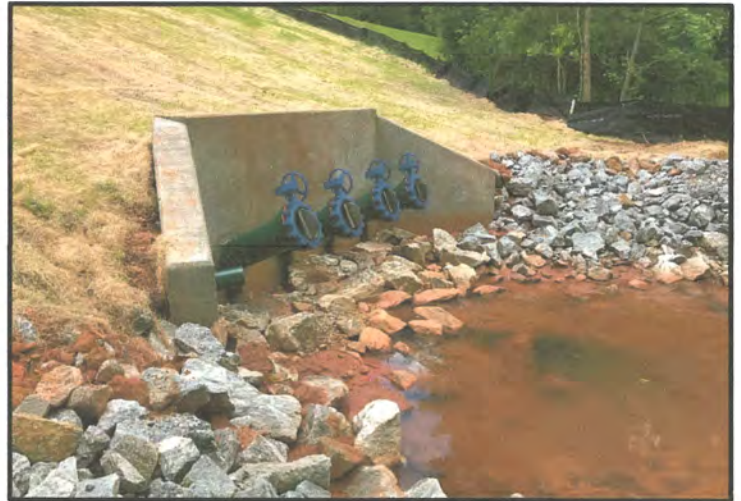
Figure 3 Typical Figure of Siphon Outlets with Butterfly Valves (NOT ACTUAL FIGURE OF BOB MITCHELL LAKE DAM)
